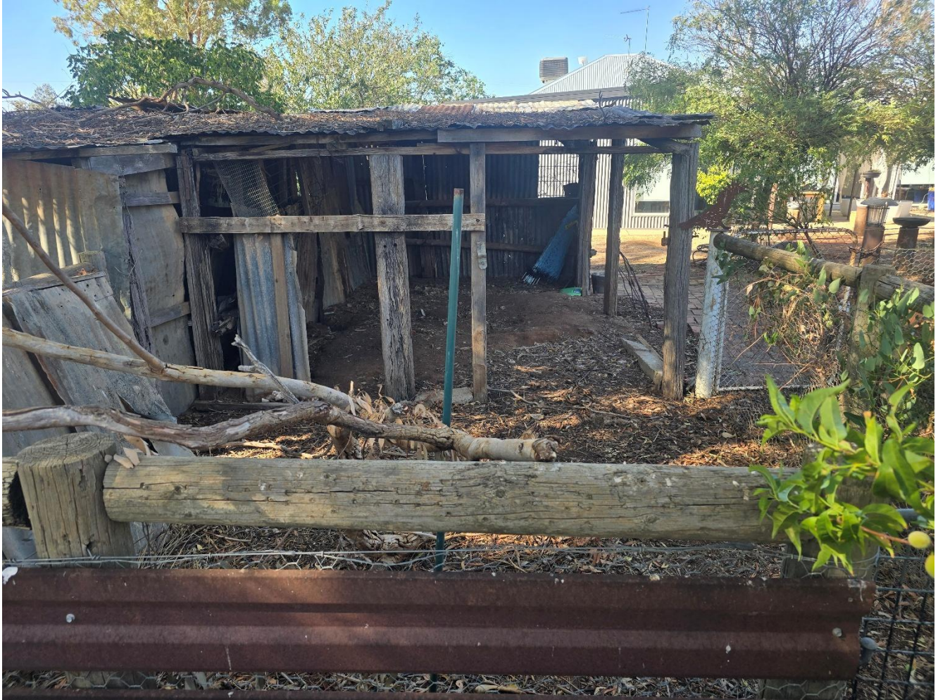
Site Photo 2 – BH2 Looking South (20/02/2026)
