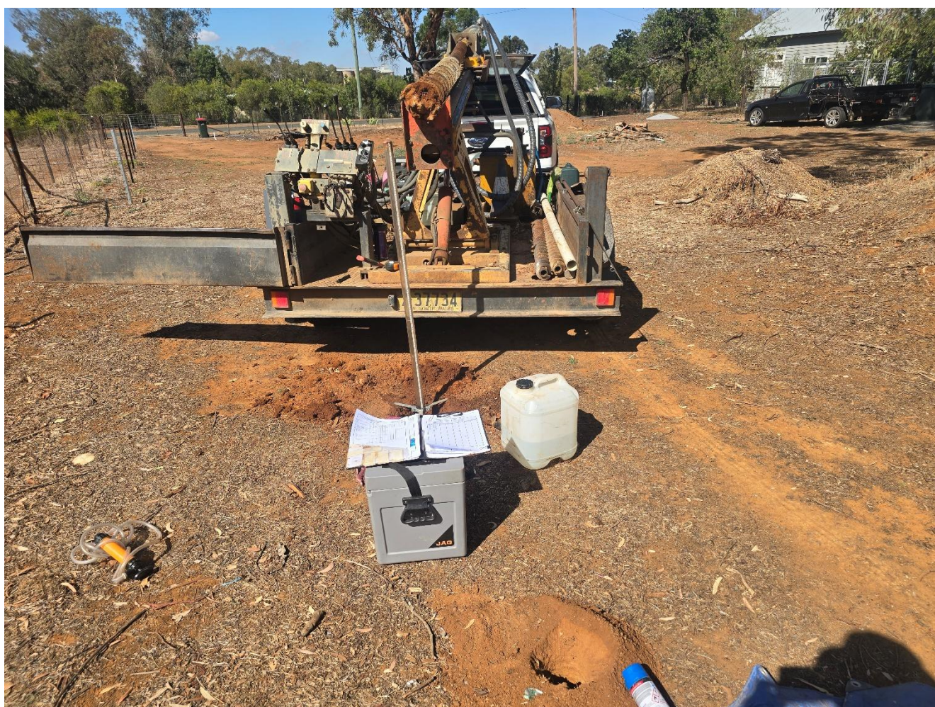
Site Photo 3 – BH3 Looking South (20/02/2026)
